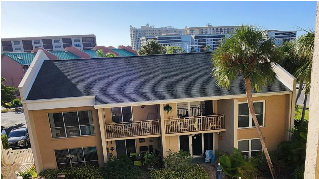
GENERAL VIEW OF ROOF
