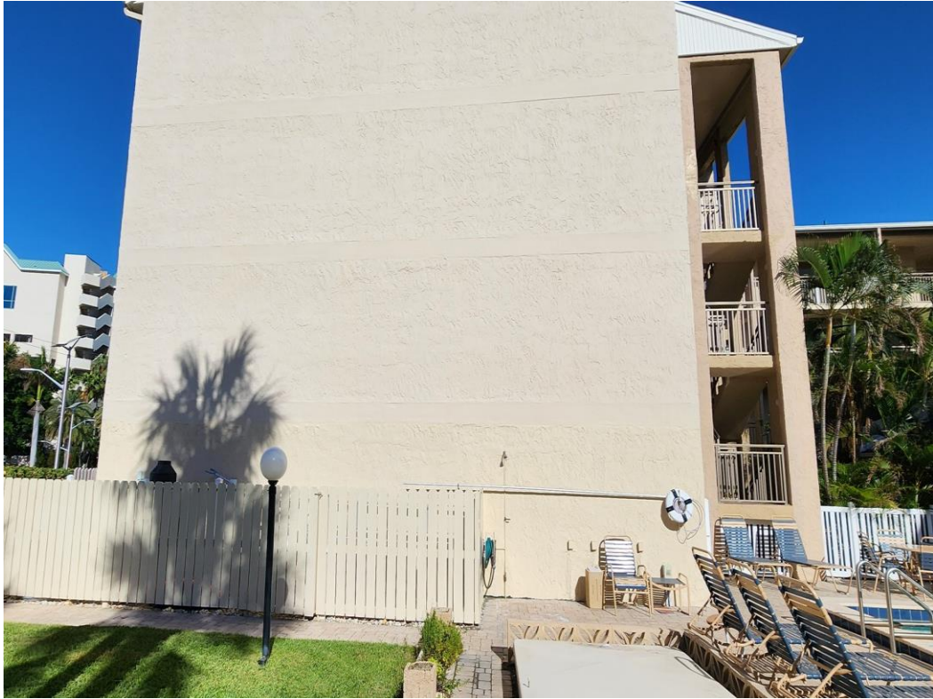
GENERAL VIEW OF BUILDING EXTERIOR FINISHES
