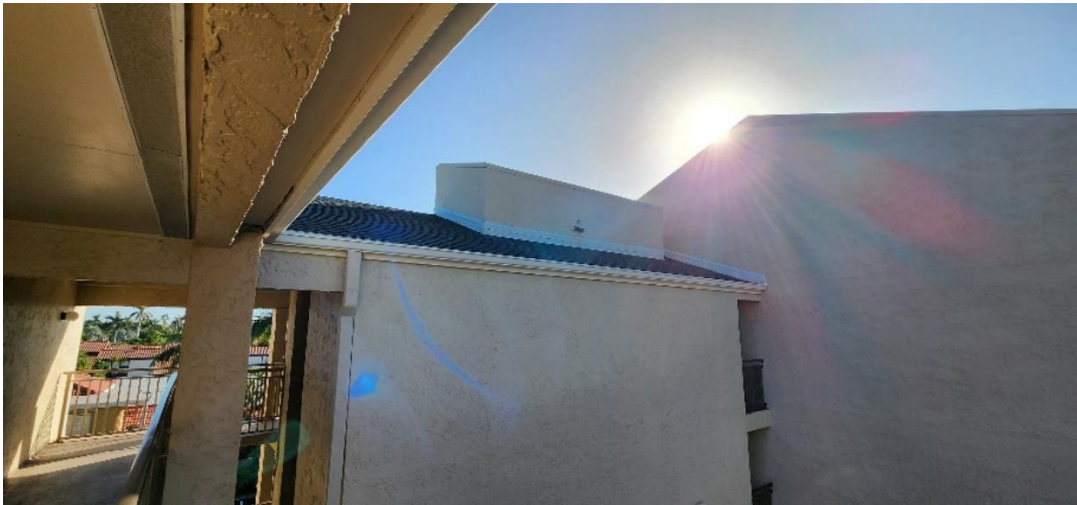
GENERAL VIEW OF STORM WATER INLET
