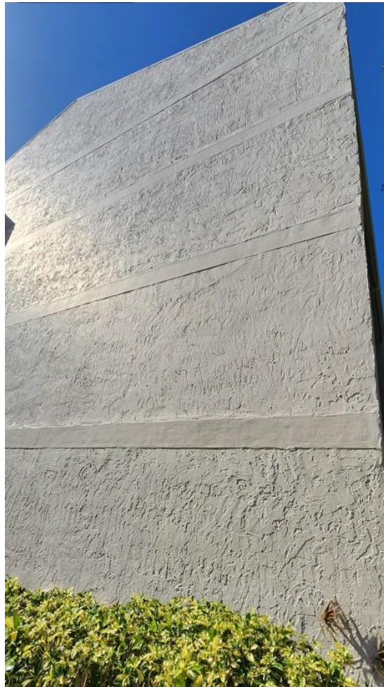
GENERAL VIEW OF BUILDING EXTERIOR FINISHES
