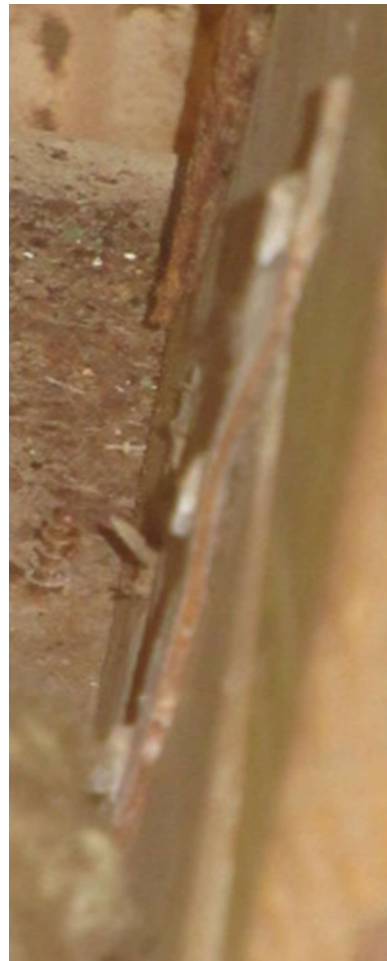
Single strap with at least 3 nails into the truss
