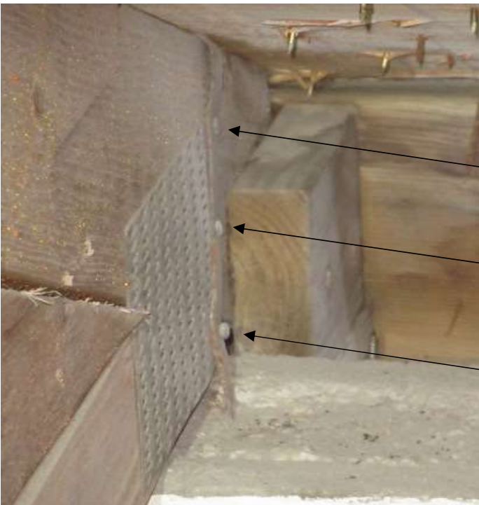
Single strap with at least 3 nails into the truss
