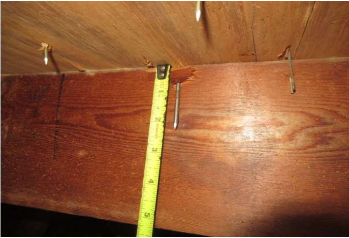
8d nails verified
